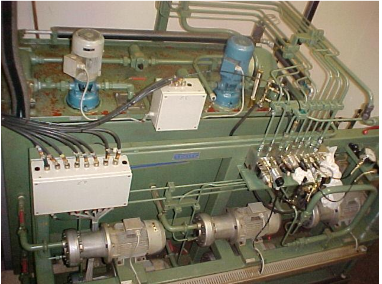
Figure 11 – Existing Hydraulic Power Pack
