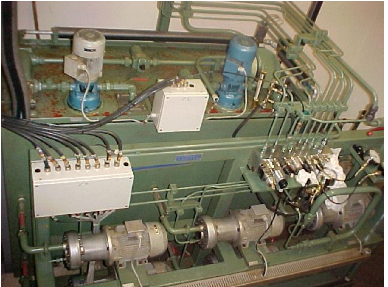
Figure 11 – Existing Hydraulic Power Pack
