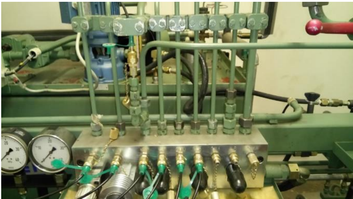
Figure 10 - Existing HPU valve block & instruments
